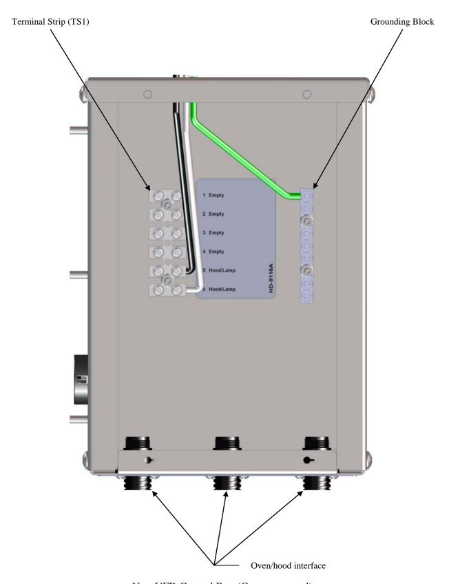
Non-VFD Control Box (Cover removed)
