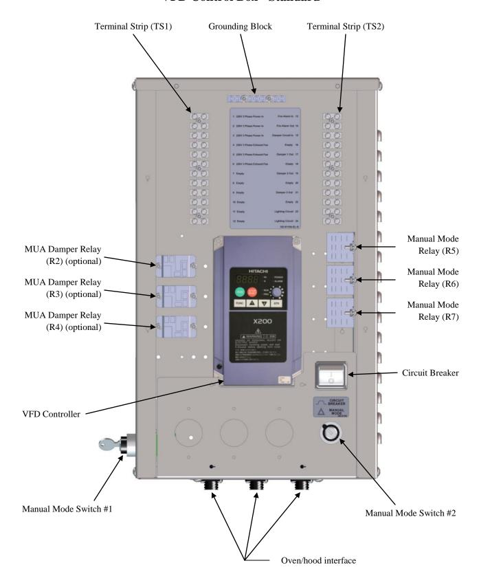
VFD Control Box (Cover removed)
