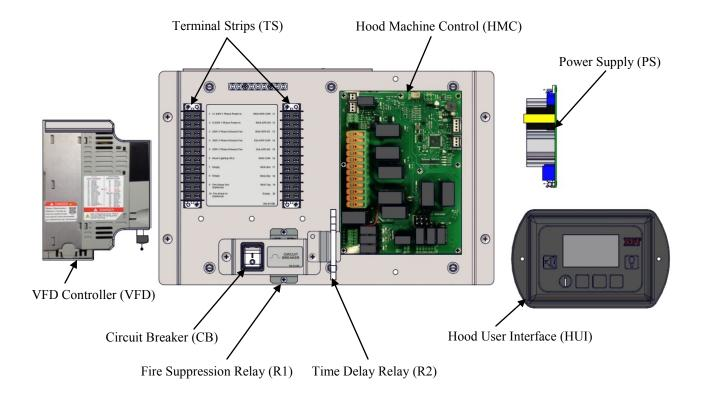
VFD Control Box (Cover removed)
